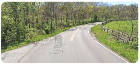
At left, superelevation on the roadway and rutting on the shoulder contribute significantly to ponding water on the inside of the curve.
