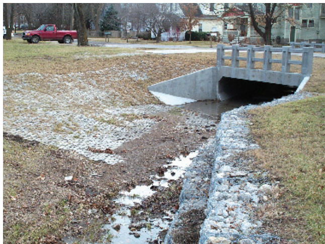
Cellular concrete mat used to stabilize banks in a highly erodible silty loam soil. Double- or triple-seed these applications immediately after installation. Mulch might be needed to support seeded areas until grass is established.
