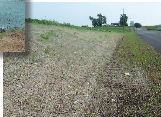
Seed ditches immediately after construction. Use mulch, netting, or erosion control blankets to protect newly seeded areas.
