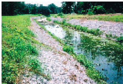
Gabion mattresses can replace turf mats in high-flow, high-velocity channels. Mixing mulch and soil into the rock can help support vegetation for a “greener” look.
