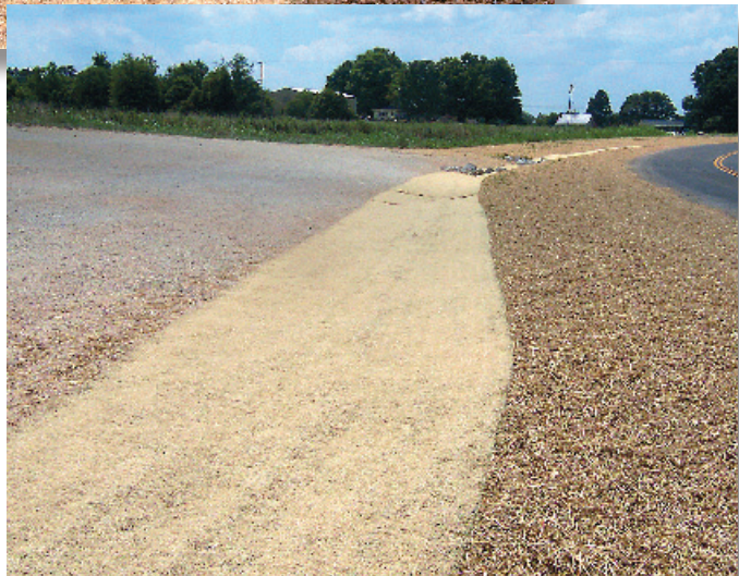
When using blankets and mats, make sure product has good soil contact throughout the ditch. Use plenty of staples to protect against surge flows during heavy rains. Blankets and mats are extremely vulnerable before seed germination, and can be dislodged by high-velocity flows if stapling is insufficient.
