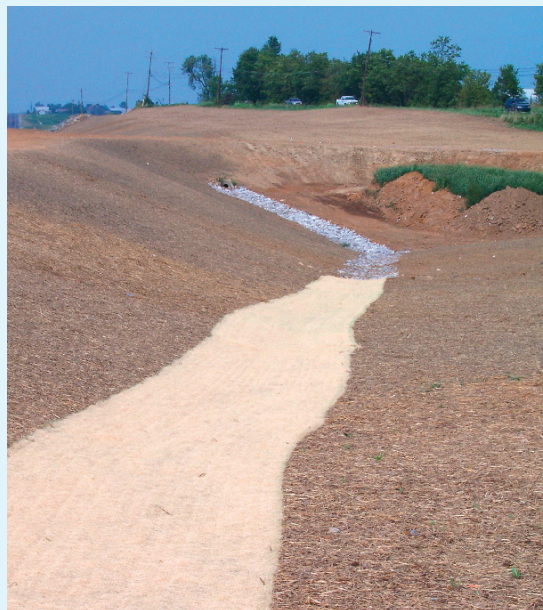
Good construction of drainage ditch, with riprap liner for steeply sloping section (background) and erosion control blanket over triple-seeding in flatter area. Ditches should be stabilized or seeded and mulched immediately after construction.
