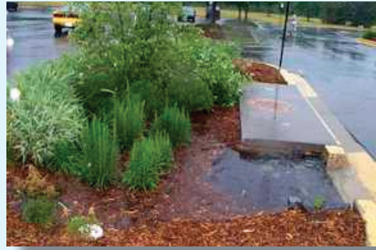
Low impact development design seeks to capture and infiltrate runoff close to the source area. Small, strategically placed "rain gardens" and other dedicated and managed infiltration sites reduce runoff volumes and remove potential pollutants.
