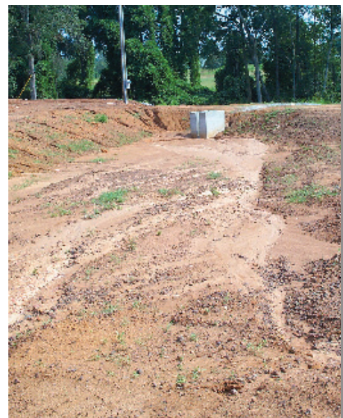
This shows a very well designed detention basin, featuring long flow path between inlet and outlet and V-notched outlet riser, which provides longer detention times for low flow events while still accommodating larger storms. Operation of this basin during the construction phase, however, is very poor. Note the lack of grass on sidewalls; no temporary dike in front of the outlet. This basin appears to be filling rapidly and requires sediment removal. For best results, seed and mulch basins immediately after construction, and modify the outlet to achieve 1 to 2 days of drain-down time after storm events.
