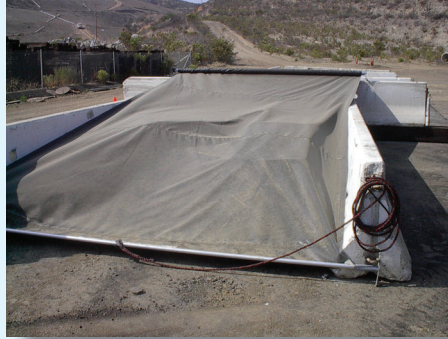
Keep construction sites well-graded, clean, and store materials properly to eliminate contaminated runoff. Wash water, fuels, and other potentially hazardous liquids should be managed appropriately.
