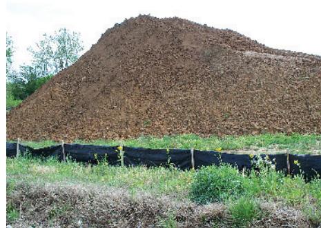
This is a good location of topsoil pile on flat, grassy area and good use of a silt fence to protect nearby creek (foreground).
